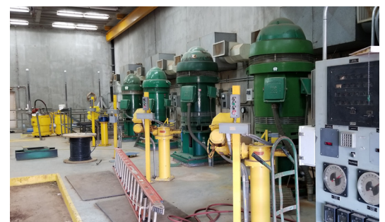
Waurika Lake Pumping Station
