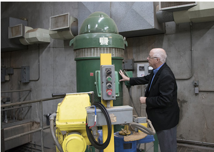
Dave Taylor Checks Pump at Pump House
